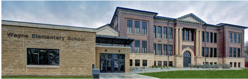
Fig. 3.2.2: Exterior front facade showing 1923 Building and 2010 Addition, 2013
